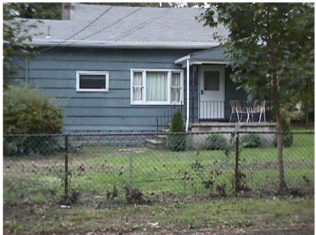
40 Hobson Street was acquired before Floyd hit. The debris line on the fence shows floodwaters were 2 1/2 feet deep.
