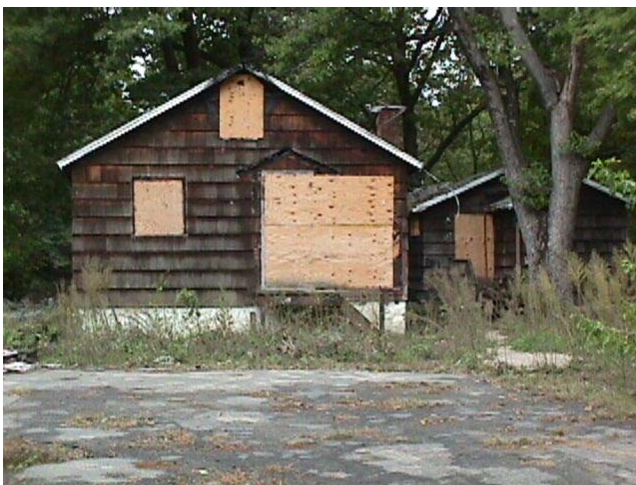
The former owners of these vacant houses on Fayette Street wisely chose to move from the Passaic River floodway.
