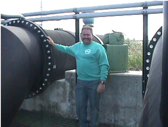
Mike Monforte, Little Ferry Department of Public Works, at the new Losen Slote Pumping Station. The new system easily handled waters from Hurricane Floyd and saved many residences from flooding.
