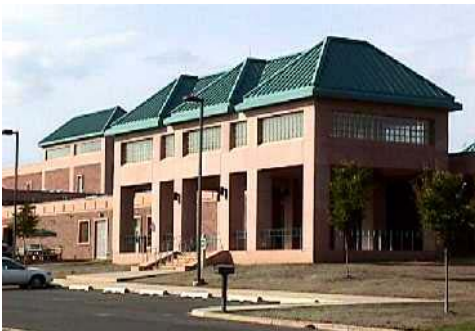
The state-of the art Elizabethtown Canal Road Water Treatment Plant cost approximately $100 million.
