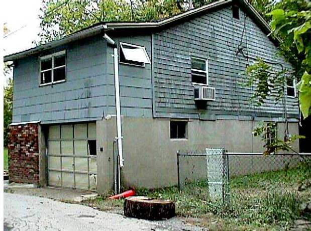
The building at 17 Island Street, acquired under the NJ Blue Acres Program, will soon be demolished. Note the high water mark at four feet on the garage door.
